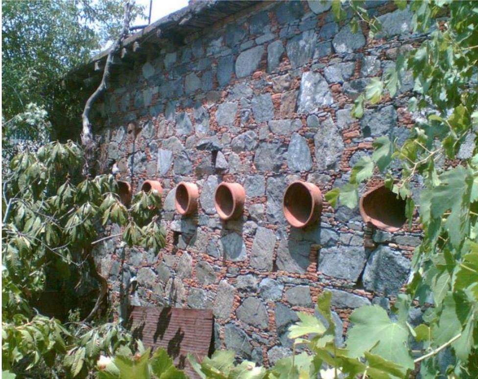
**Fig. 5:** Traditional horizontal, open at both ends, clay beehives embedded in a house wall in the village of Agros, Cyprus (Photo: L. Eleftheriou).
